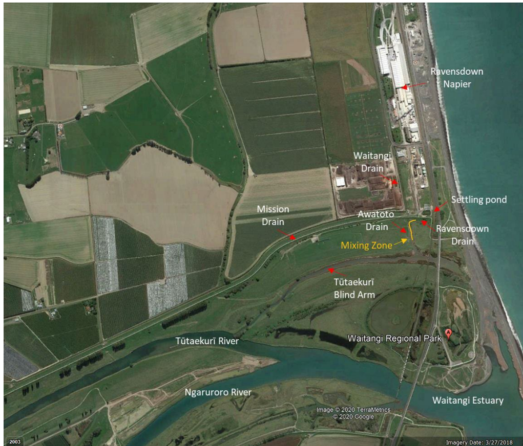
Figure 4: Current Napier Works stormwater and process water discharge receiving environment and associated waterways. 8
