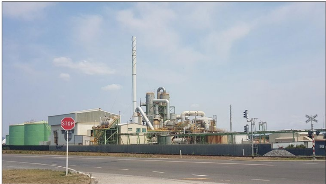
Figure 12: View of Acid Plant from State Highway 51.
