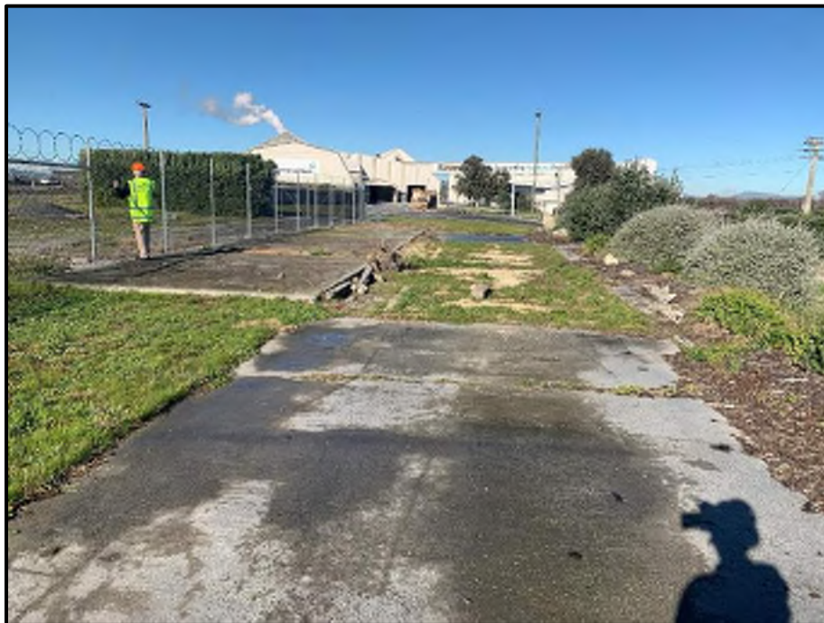
Photograph 20: Remnants of the Former Weighbridge South of the Truck Depot
