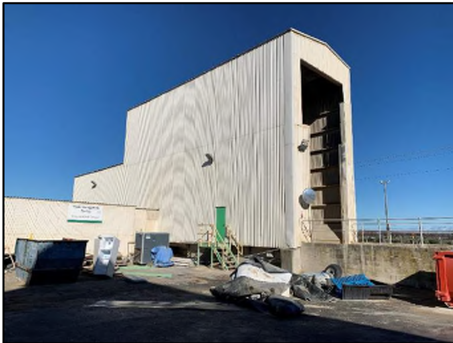
Photograph 32: View of the Intake Area Towards the South of the Site
