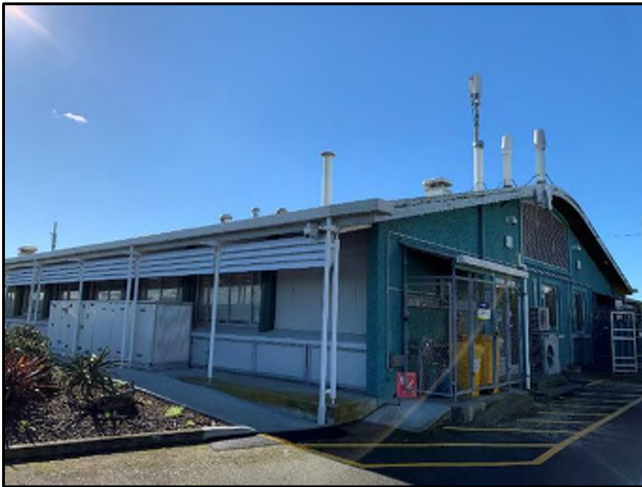
Photograph 6: General View of the Commercial Laboratory on Section 62 Block I Clive SD and Section 43 Block I Clive SD
