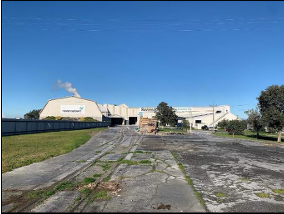
Photograph 21: Former Railway Lines in the North of the Site
