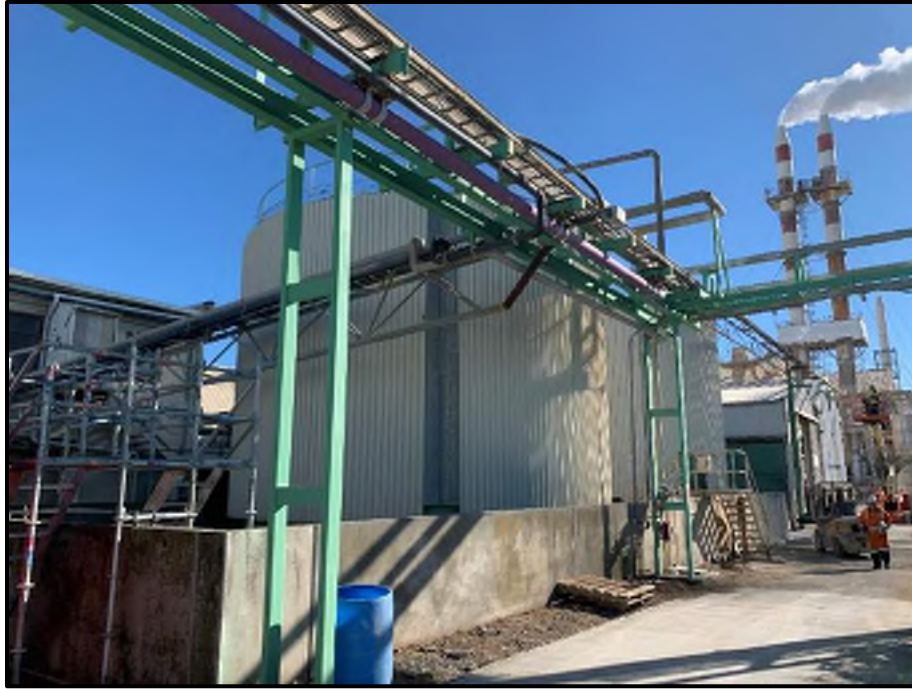
Photograph 31: View of the Bunded Acid Tanks South-East of the Above Garage
