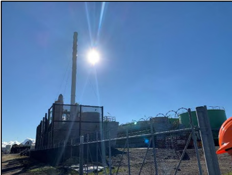
Photograph 16: General View of the Cooling Towers on Part Section 32 Block I Clive SD
