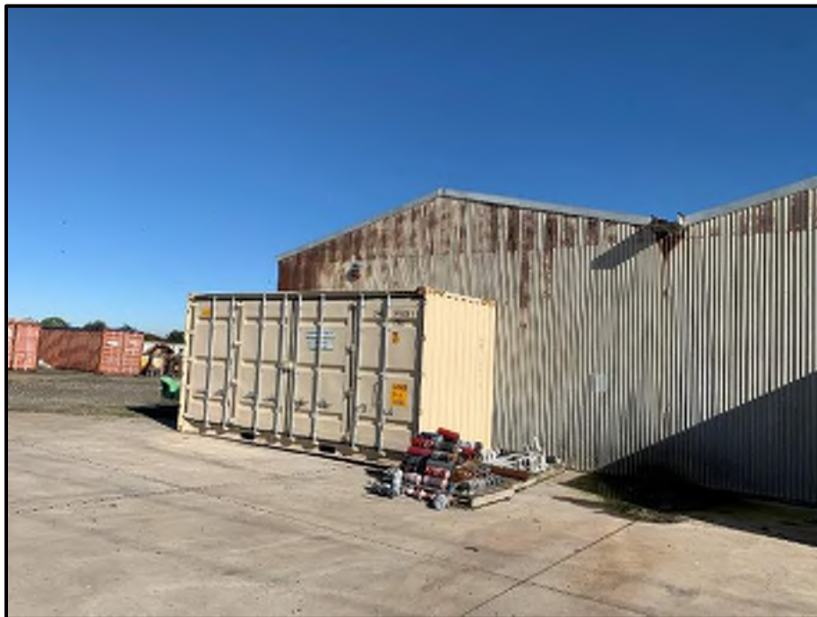
Photograph 10: Example View of the Shipping Containers used as Inventory Stores External to the Engineering Store on Lot 2 DP 16060
