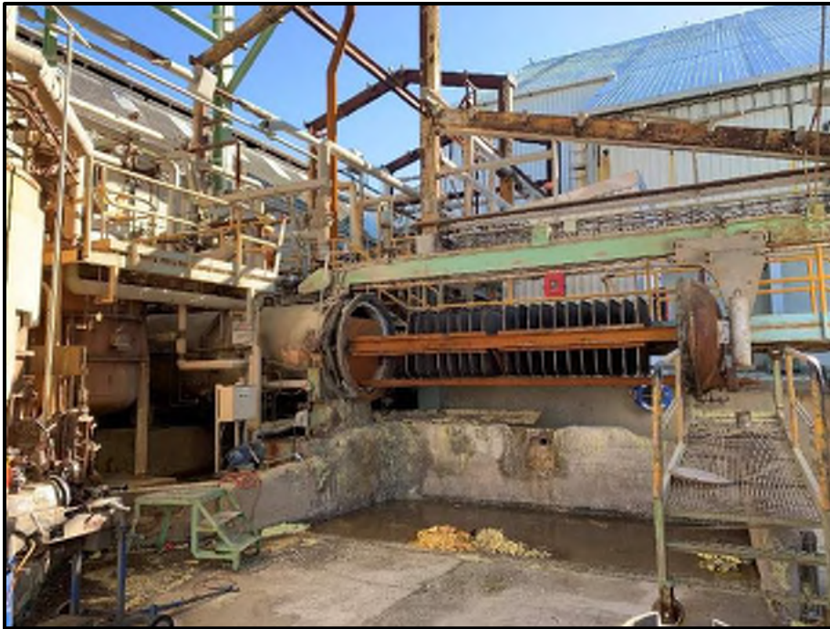
Photograph 36: View of the Sulphur Melter Towards the South of the Site
