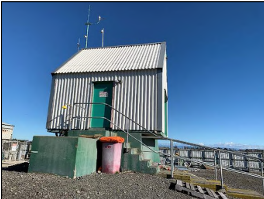
Photograph 8: View of the Pumphouse on Lot 2 DP 16060
