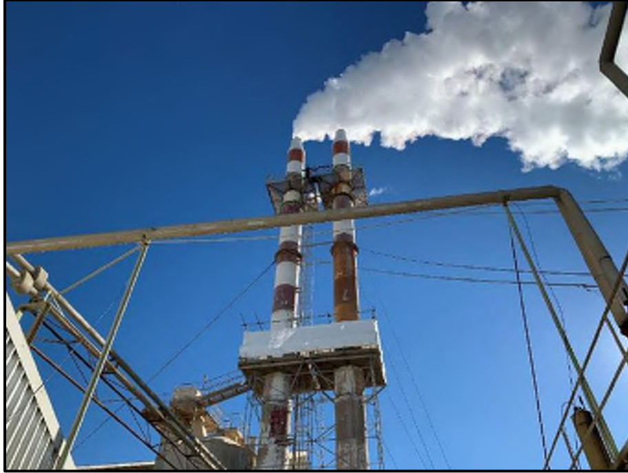
Photograph 27: View of the Stacks South of the Manufacturing and Granulation Building
