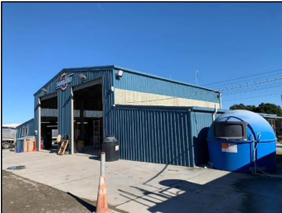
Photograph 18: General View of the Workshop at the Truck Depot in the North of the Site
