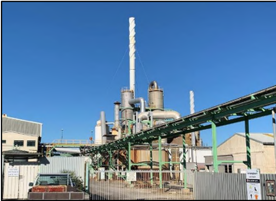
Photograph 14: General View of the Acid Plant on Part Section 32 Block I Clive SD
