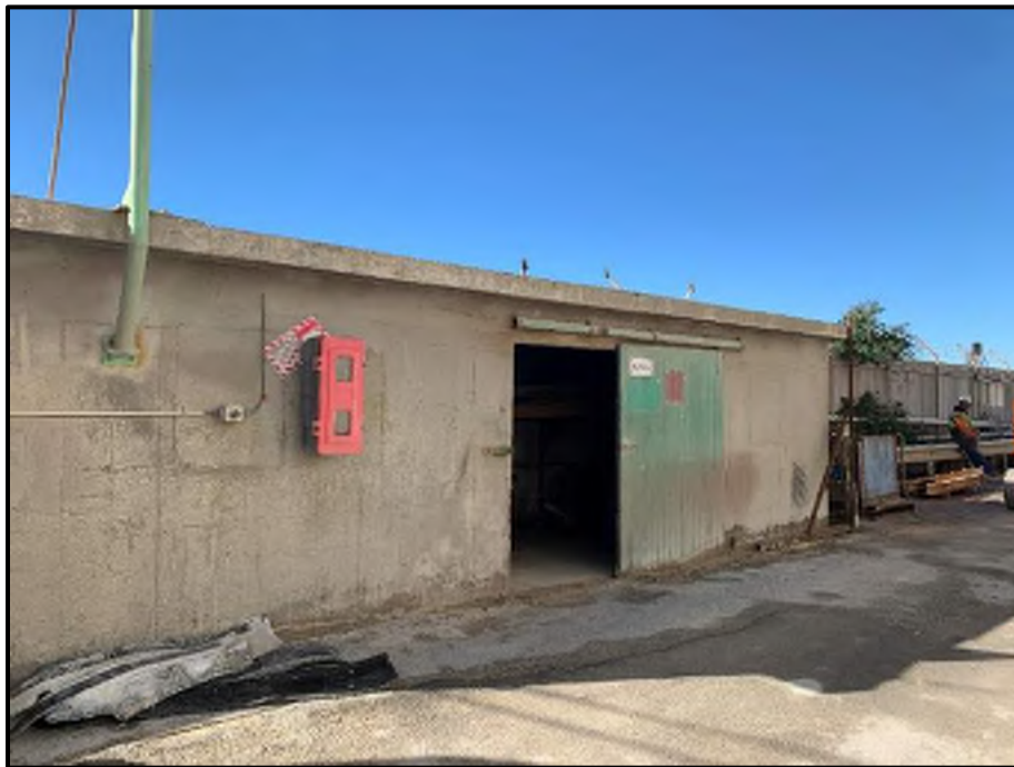
Photograph 28: View of the Disused Former HazChem Store South-East of the Manufacturing and Granulation Building
