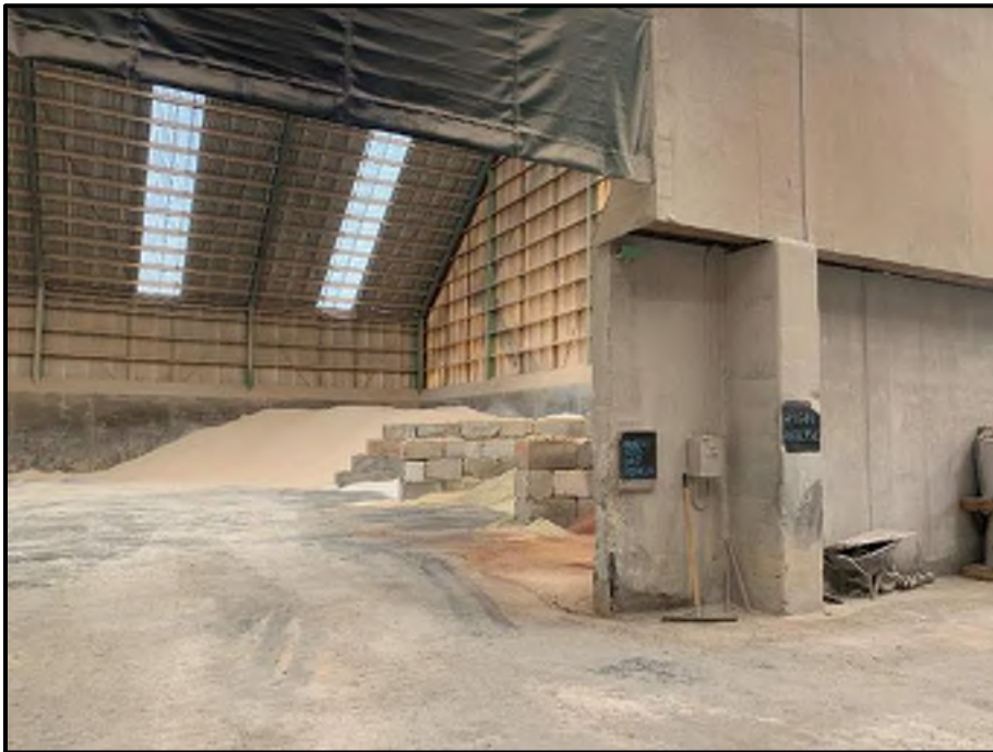
Photograph 24: Internal View within No 1 Super Store
