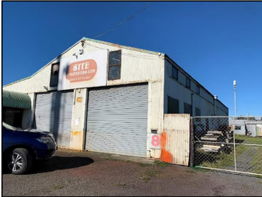
Photograph 3: General View of the Current Engineering Workshop (Former Truck Shed and then Tannery) on Part Section 43 Block I Clive SD
