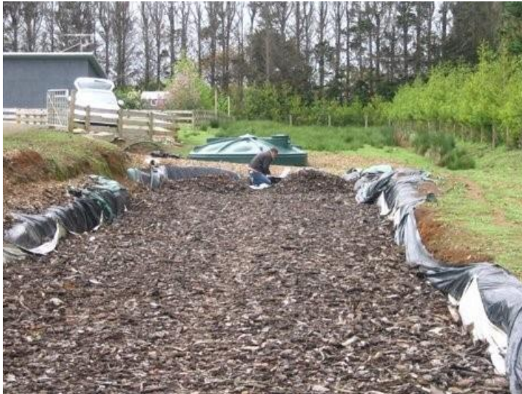
Figure 8 Wood chip bioreactor (Queensland Government)
