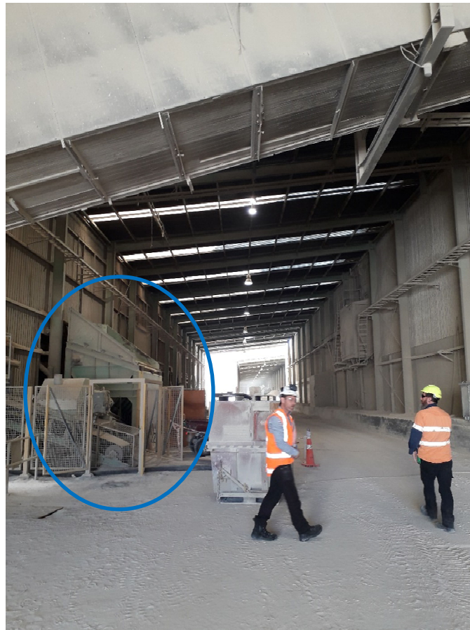
Photo 3 Storage Shed Corridor Showing Location of the Rock Intake Hopper
