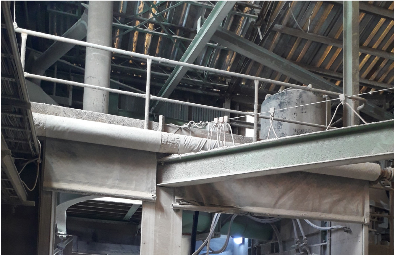
Photo 9 Curtains for the Mixer
