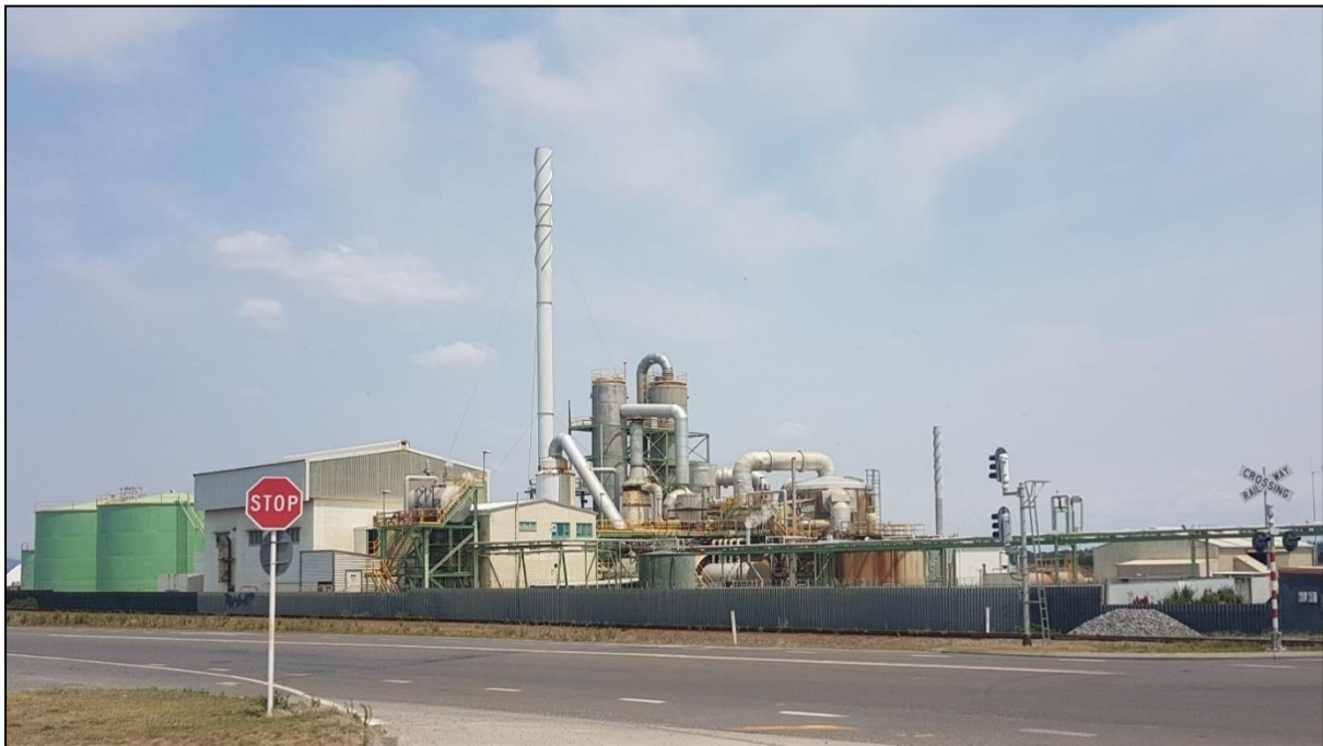
Figure 2.5: View of Acid Plant from State Highway 51.
