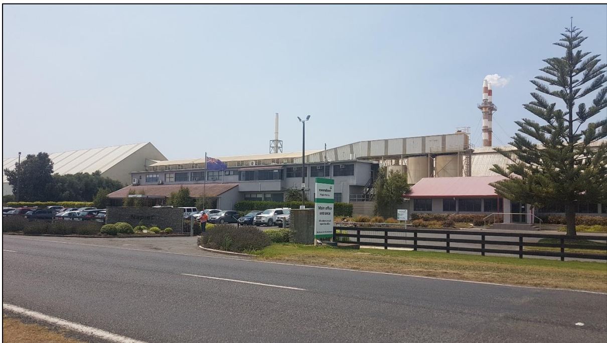
Figure 2.7: View of the Manufacturing Plant looking from Waitangi Road across the site office. The stacks to the right are the existing Den Scrubber stacks and the stack in the distance to the left is the existing Hygiene scrubber stack.
