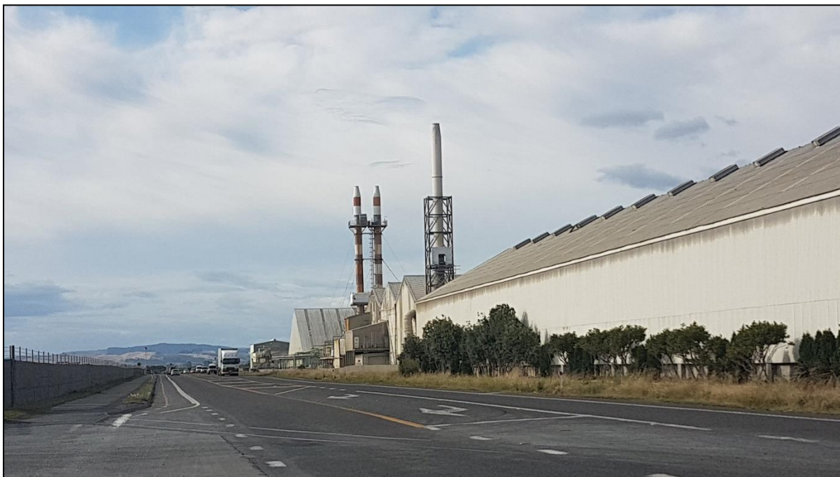
Figure 2.8: View of the Manufacturing Plant looking from SH51. The stacks in the background are the existing Den Scrubber stacks and the stack in foreground is the existing Hygiene scrubber stack.
